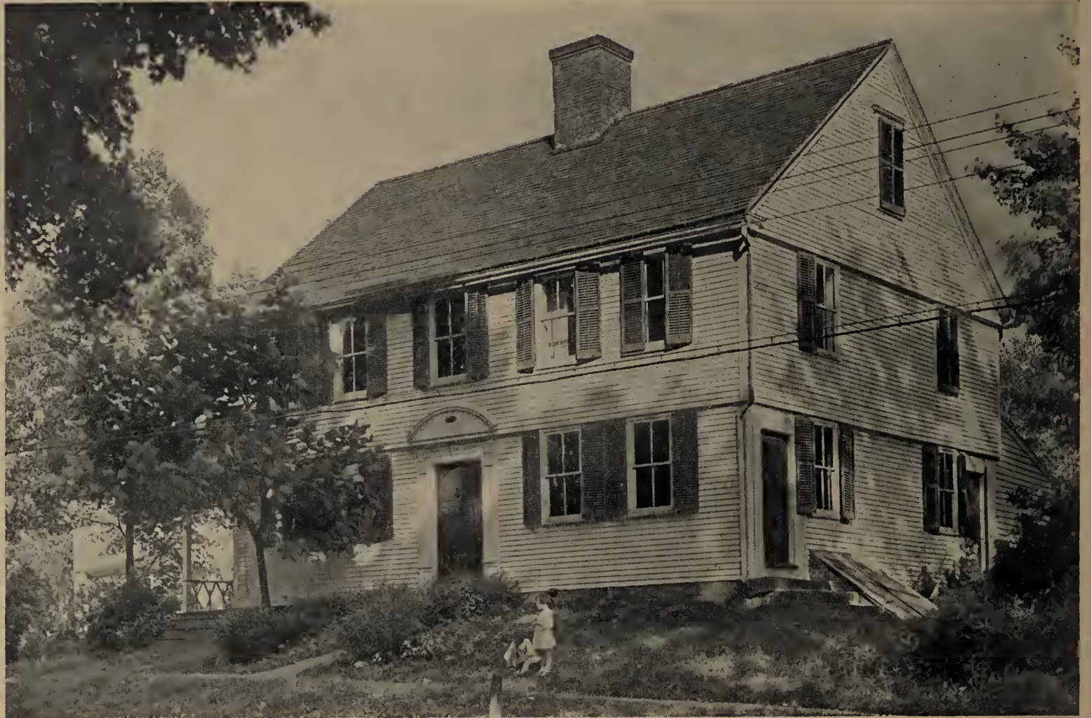
THE JOHNSON HOUSE, FARMINGTON, CONNECTICUT Built in 1690
