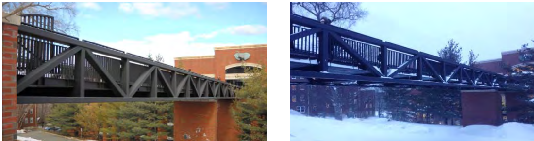
Fig. 1 South view of Dowling Hall Footbridge
