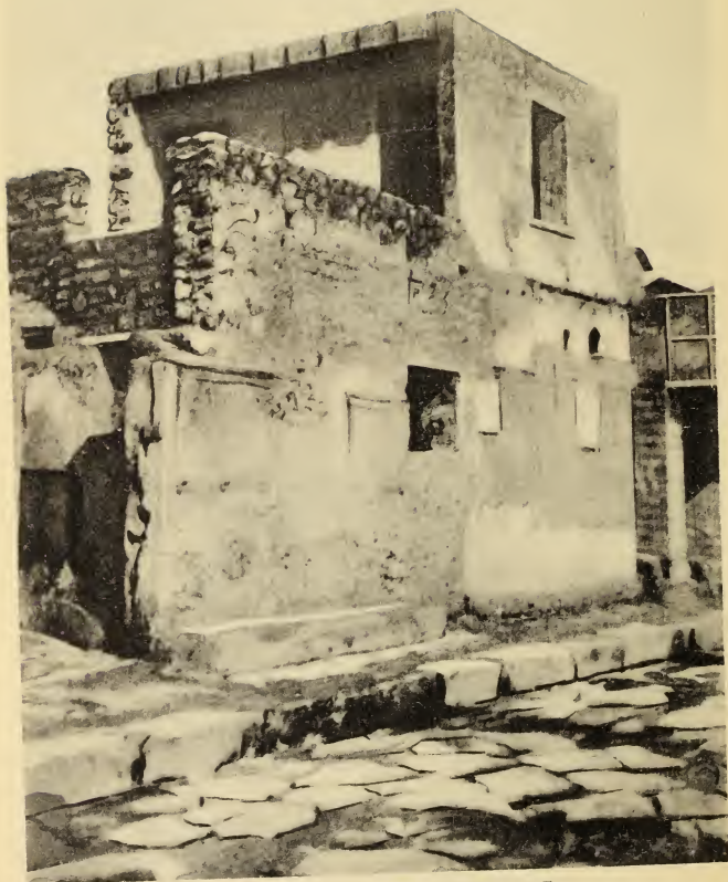
LA CASA COL PIANO SUPERIORE UPPER STORY OF A HOUSE IN THE IS. IV REG. III
