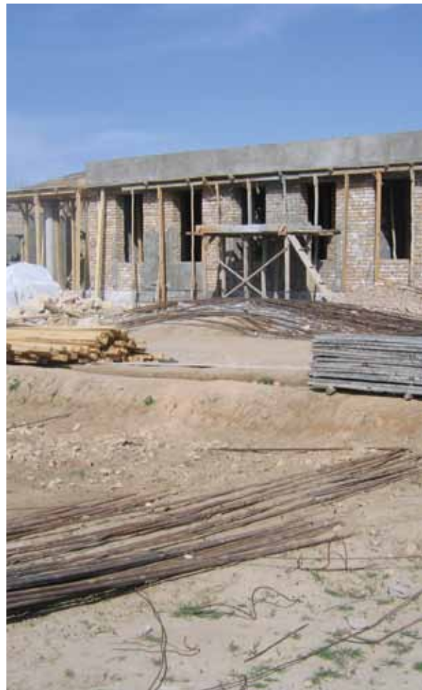
School construction in Khwoja Namusa, Pashtun Kot
