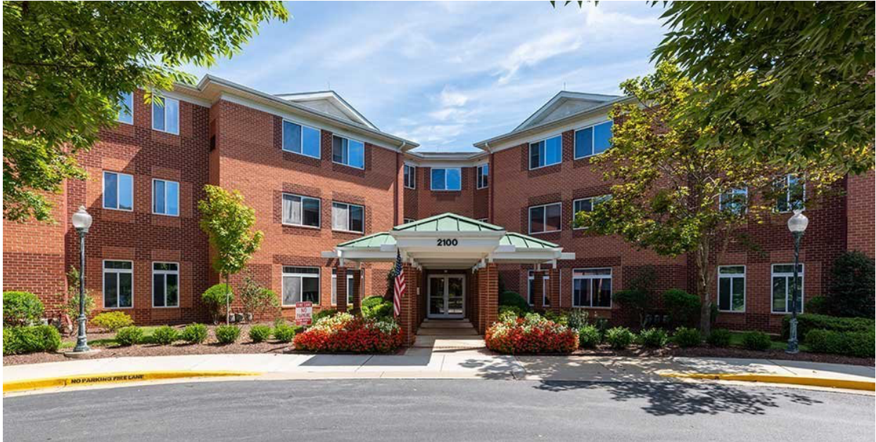
Fig. 2: Entrance to the Andrew Kim House. Image Credit: Victory Housing.
