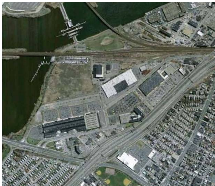
Figure 14: Aerial View of Current Assembly Square Mall
