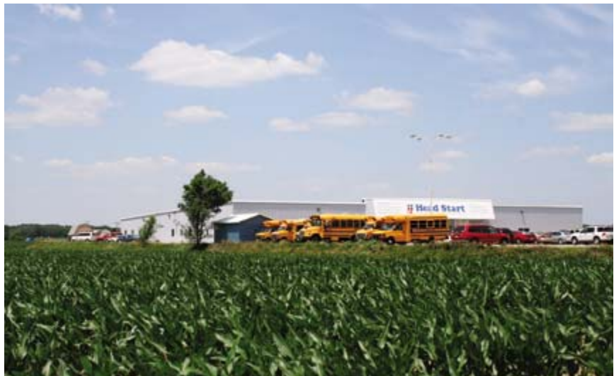
Figure 8: View of Head Start Center from Surrounding Cornfields
