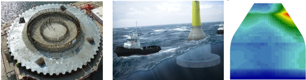
(c) SeaTower Gravity Base Offshore Wind Support Structure with Finite Element Model 6
