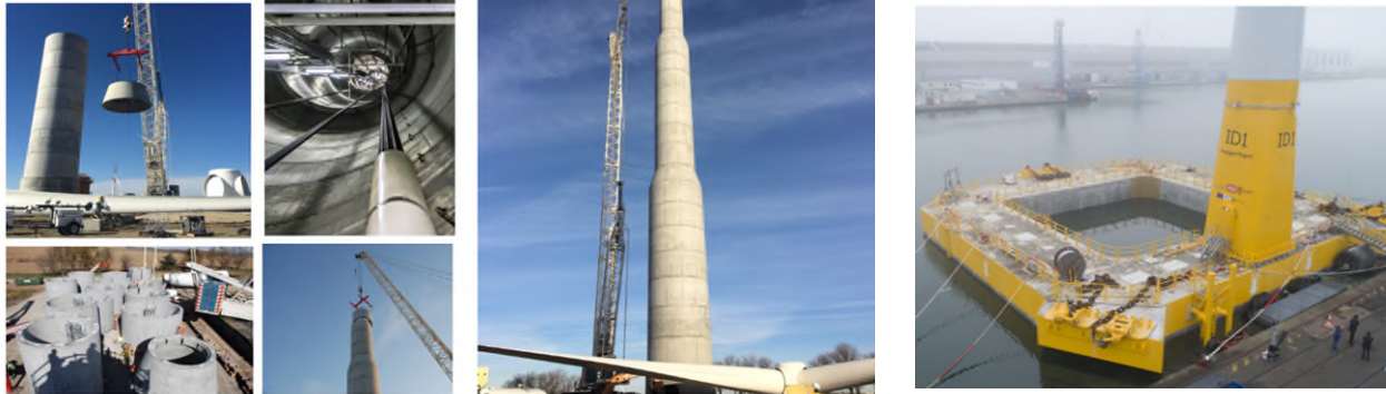
(a) Wind Tower Technologies Precast Tall Tower Solution 4 (b) Floatgen Offshore 5 Foundation
