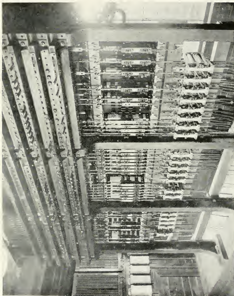
INTERIOR OF "ALL-ELECTRIC" INTERLOCKING FRAME ("CREWE" SYSTEM), L. AND N. W. R.
