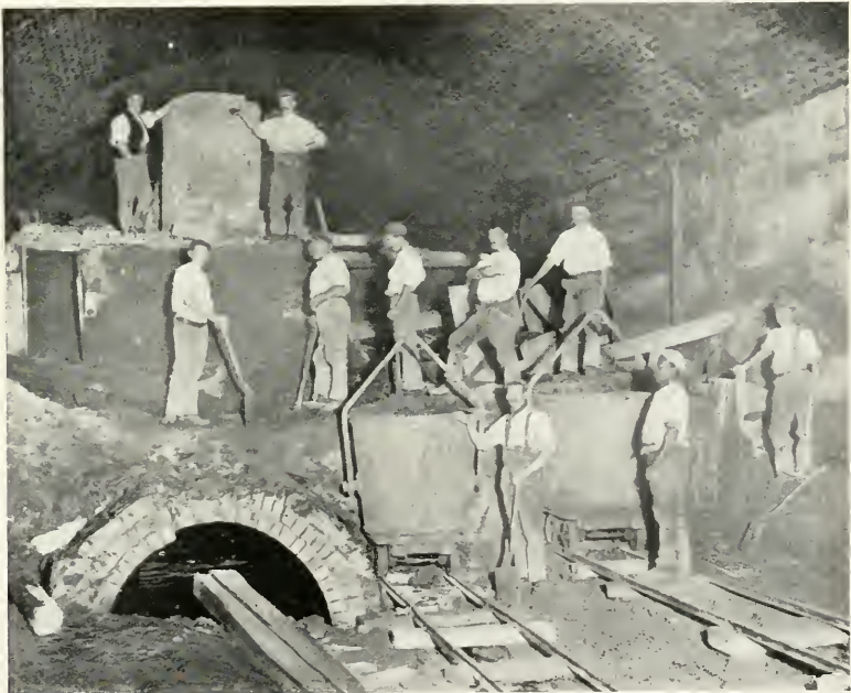
WITH "CUT AND COVER" THE WORK IS DONE FROM THE TOP. FINALLY THE REMAINING EARTH, VULGARLY CALLED THE "DUMPLING," IS REMOVED.
