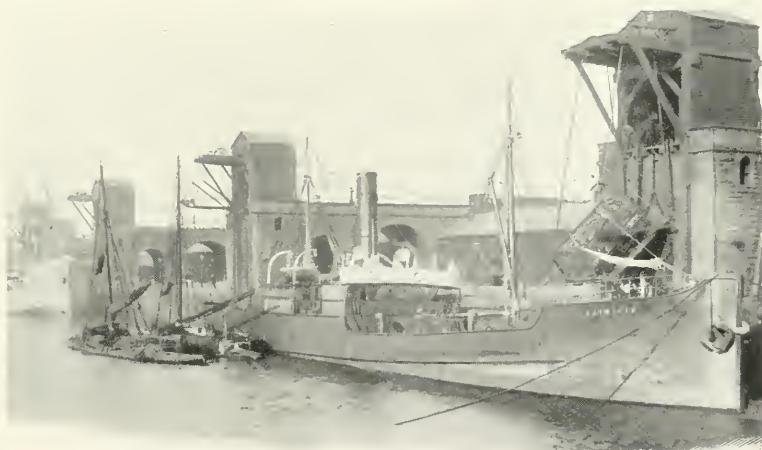
COAL-TIPS AT GARSTON DOCKS, NEAR LIVERPOOL, L. AND N. W. R.
