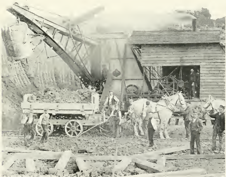
AT THE COMMENCEMENT, HORSES PULLING "TIP-WAGONS" ARE WORKED BETWEEN THE FACE OF THE EXCAVATION AND THE "TIP-HEAD" WHERE AN EMBANKMENT IS BEING FORMED.
