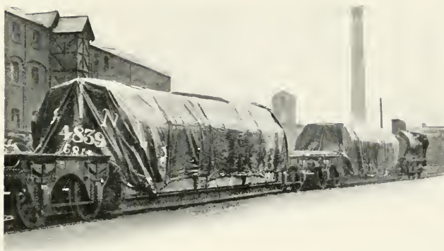
CONVEYANCE OF GLASGOW DISTRICT SUBWAY CABLE, 7 MILES LONG, BY L. AND N. W. R.
