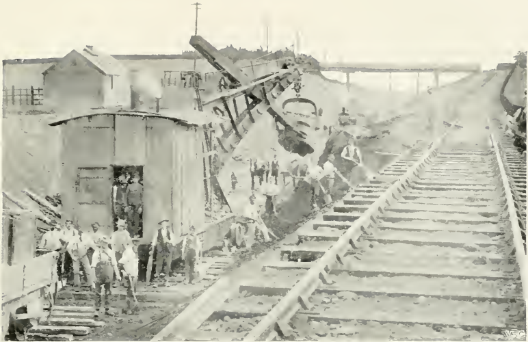
THE EXCAVATION OF A NEW LINE OF RAILWAY IS COMMENCED AND PROCEEDED WITH IN SUCH A WAY THAT A TEMPORARY LINE CAN BE LAID DOWN AS EARLY AS POSSIBLE. ON NEARLY ALL JOBS IT IS CUSTOMARY TO BRING A "STEAM NAVVY" ON TO THE WORKS.
