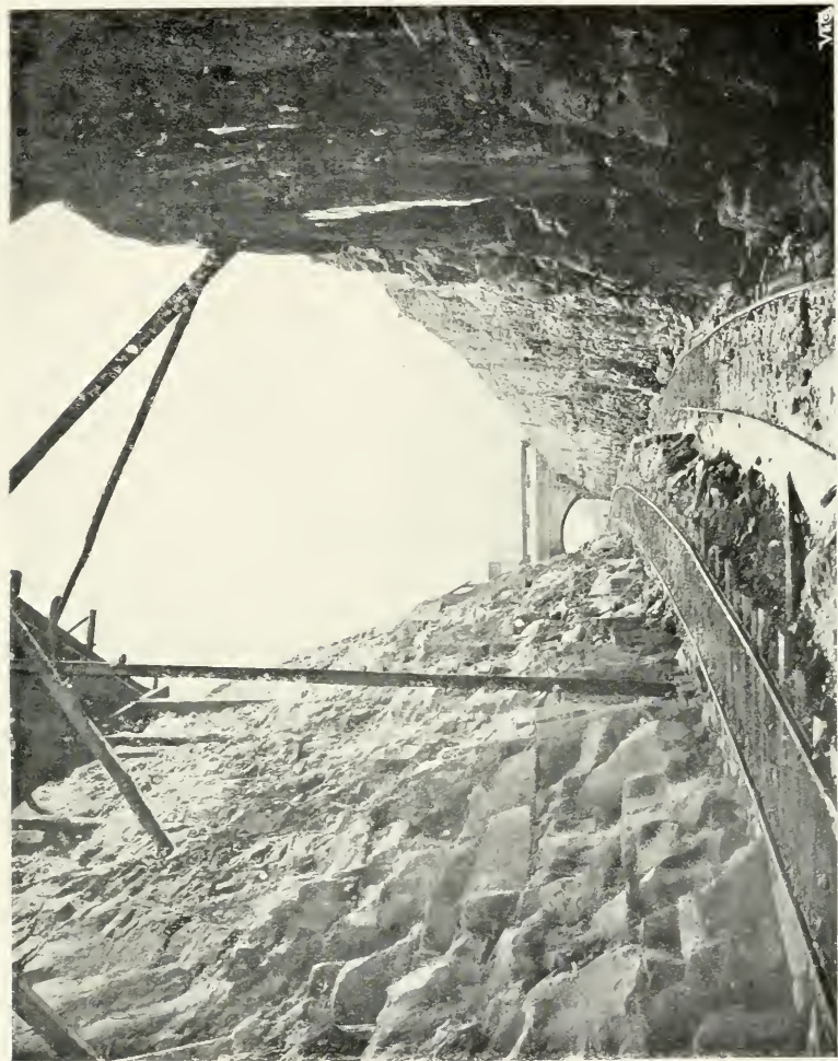
IF MUCH ROCK HAS TO BE REMOVED, BLASTING IS USUALLY THE METHOD EMPLOYED FOR DISLODGING IT.
