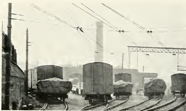
OVERHEAD CONSTRUCTION FOR WORKING GOODS TRAFFIC BY ELECTRICITY. MANORS (NEWCASTLE) GOODS YARD, N. E. R.
