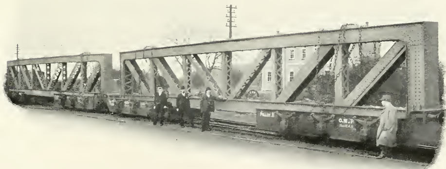
TWO LARGE GIRDERS LOADED ON G. W. R. TROLLEY-WAGONS.
