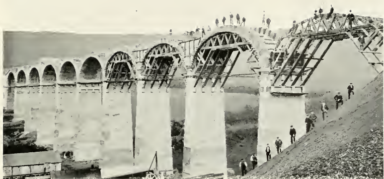
THE ERECTION OF A CABLEWAY IS OCCASIONALLY ADOPTED TO FACILITATE THE CONSTRUCTION OF A VIADUCT.
