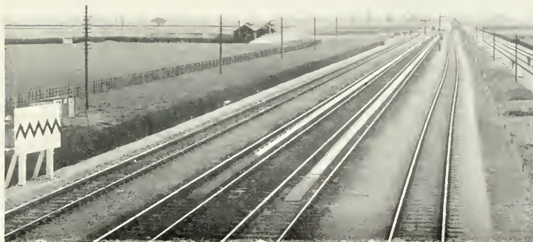
"PICK-UP" WATER-TROUGHS NEAR PETERBOROUGH, G. N. R.
