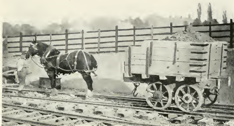
THE TRAIN IS EMPTIED WAGON BY WAGON BY A "TIP-HORSE."
