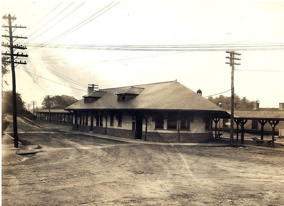
Figure 53. Old Train Depot, 1906 (Source: Andover Center of History and Culture: https://preservation.mhl.org/100-school-street )
