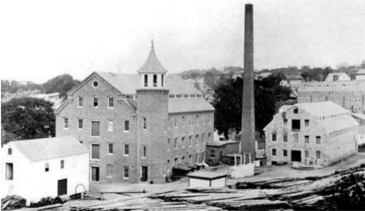
Figure 40. Smith and Dove Mill in Abbot Village, Now Dundee Park (Source: Andover Historical Society)
