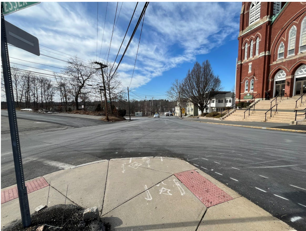
Figure 56. View of the Brook, Ridge, and Essex Intersection Looking West from the Apex of the Intersection. (Tony Collins).
