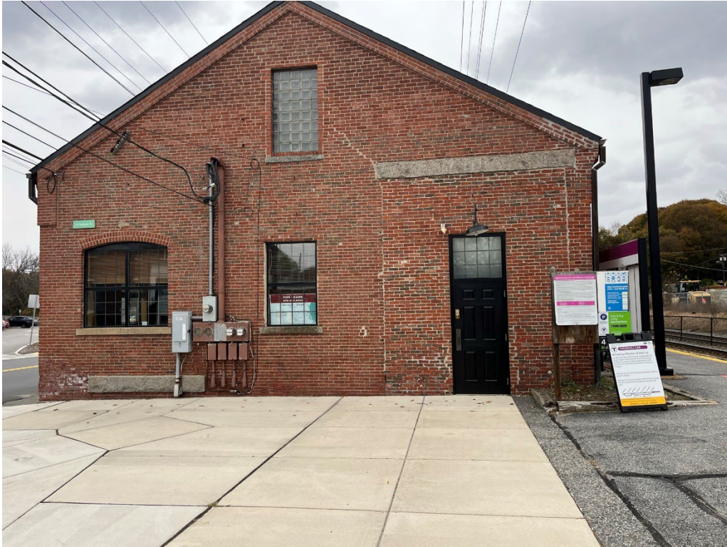
Figure 44. Old Freight Building with visible cutout of where freight cars would enter to be repaired. (Tony Collins).
