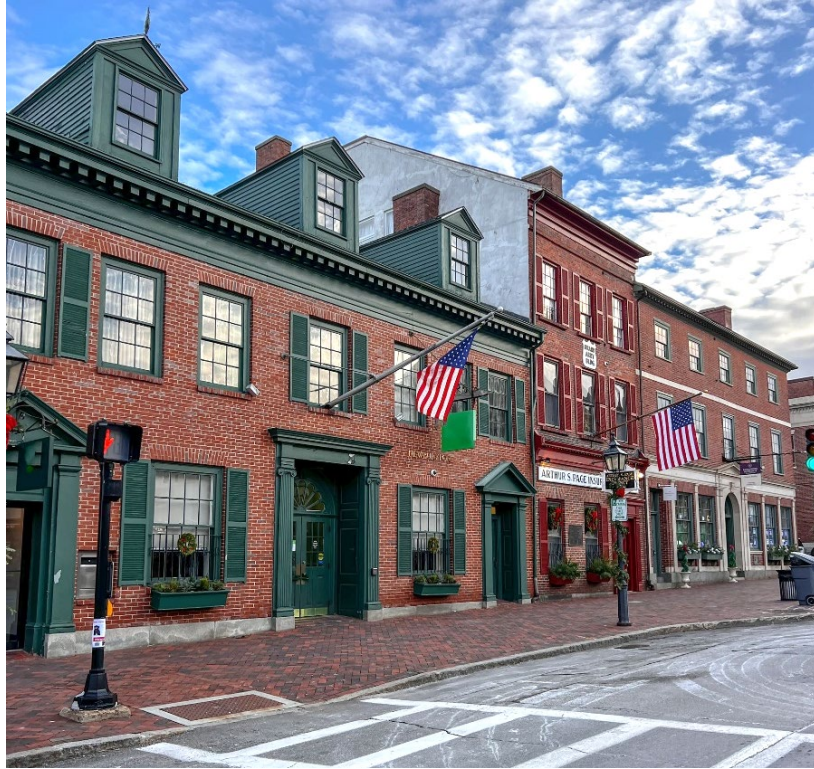
Figure 28. Human Scale, Mixed Use on State Street, Newburyport, MA (Source: Jonathan Berk)
