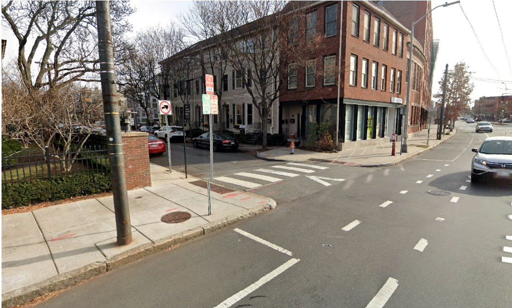
Figure 34. Continuous Sidewalk (Raised Crosswalk) Along Massachusetts Ave., Cambridge, MA (Source: Google Maps)
