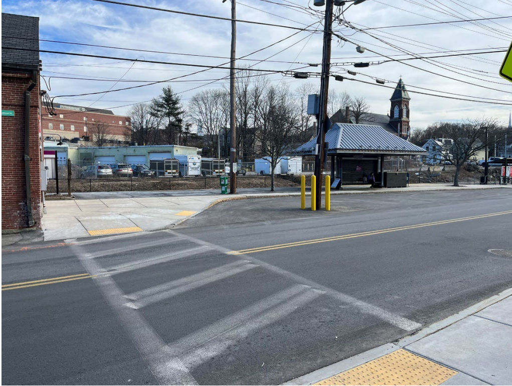
Figure 43. Crosswalk from southbound to northbound side of Railroad to the Andover Station Platform. (Tony Collins).
