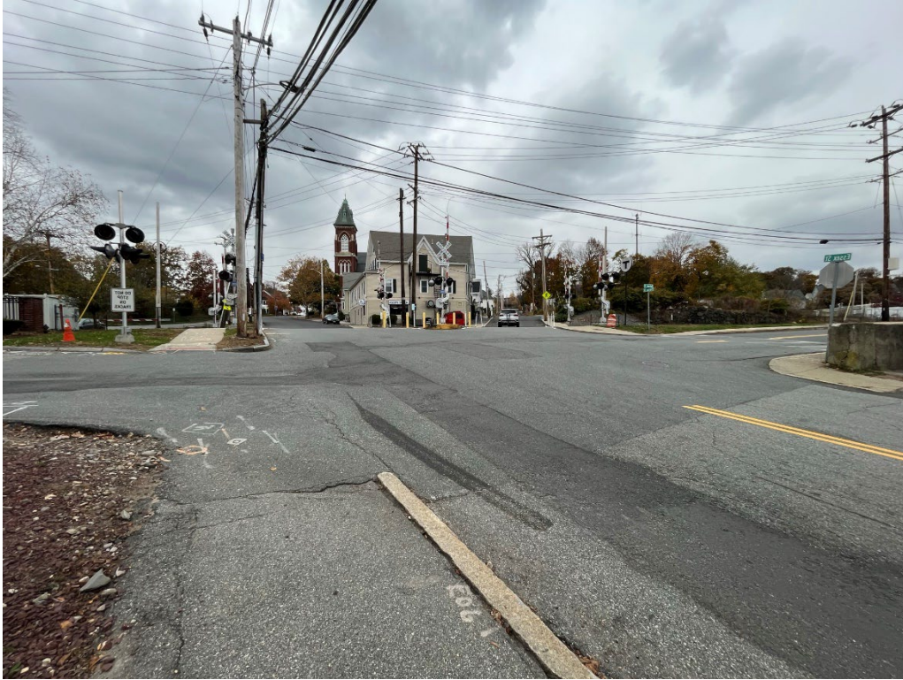
Figure 54. View of the Essex, Railroad, and Pearson Intersection Looking East on the Eastbound Side of Essex. (Tony Collins).
