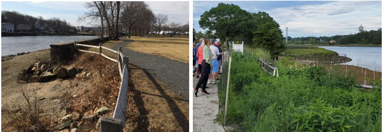
Figure 12. Nature based solutions project in Watson Park, Braintree, MA. Before (left) and after (right). The project is funded by a CZM Coastal Resiliency Grant (Town of Braintree 2022).
