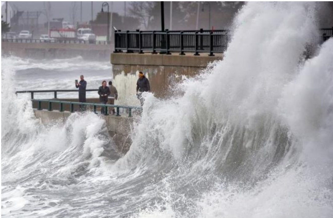
Figure 5. Seawall along Lynn Shore Drive, in Lynn, MA reducing the impact of high energy waves during a winter storm in 2021 (Garfinkel 2021).
