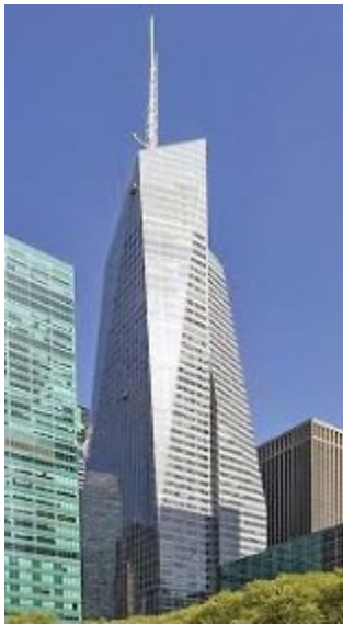
Figure 26: Bank of America Tower, NYC 2007
