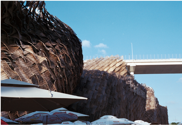
Figure 2.3. The Spain Pavilion's wicker plates undulate against its urvacous structure. In the back, the Lupu Bridge connects the two sides of the River. Photo by author.
