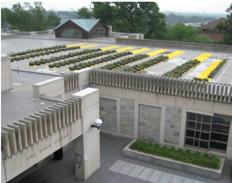
Figure 2.4 Experimental modular green roof on Tisch Library at Tufts University Medford, MA
