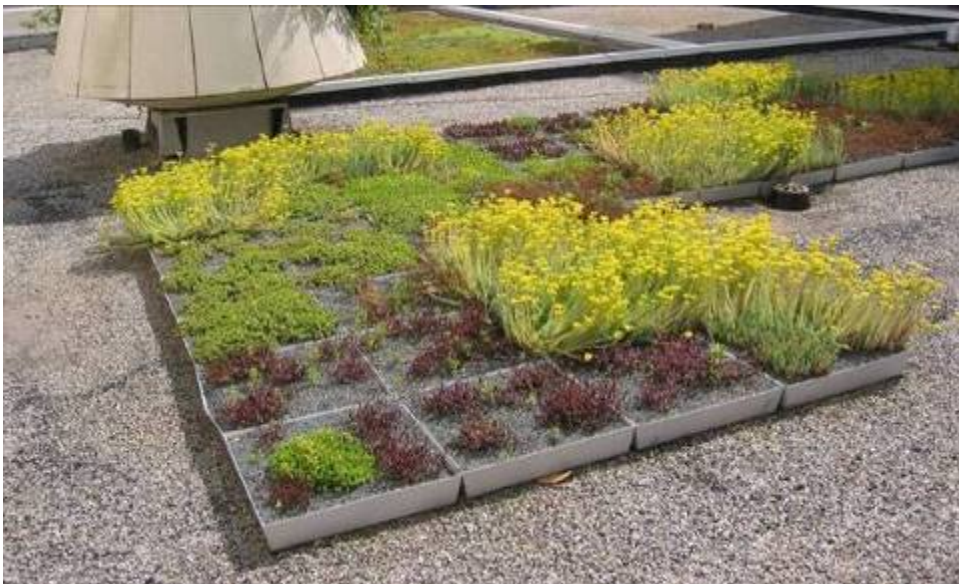
Figure 2.2 University of Georgia modular green roof system
