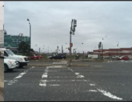
This is really wide and also needs more paint
