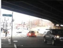
This underpass needs help
