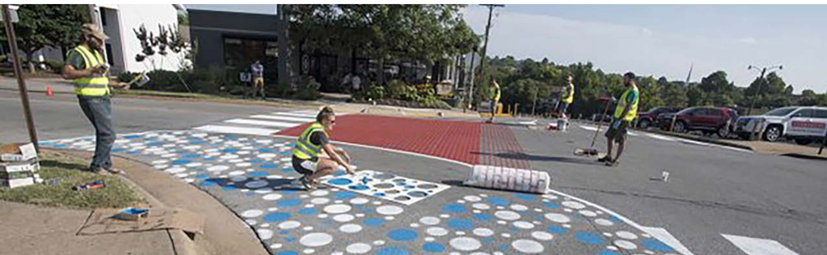
Photo: Nwa Democrat-Gazette/J.t. Wampler: Volunteers On July 23 Paint A Crosswalk And Curb Extensions At Church Avenue And Center Street In Fayetteville, Arkansas As Part Of The City's Tactical Urbanism Program.
