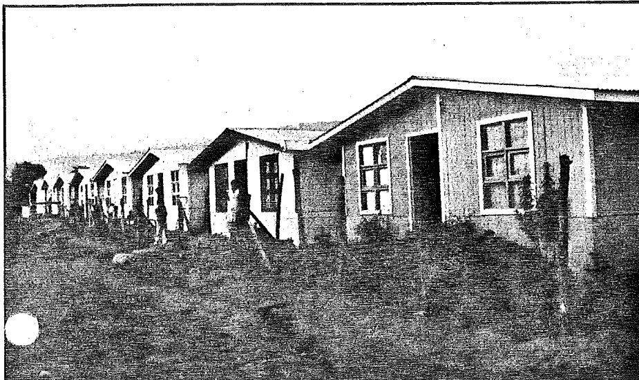
These new houses have a clean water supply now, thanks to an AID project.
