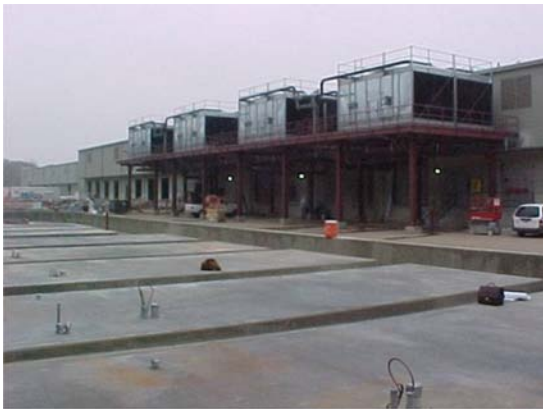
Figure 2.7 Direct cooling towers on an elevated platform.
