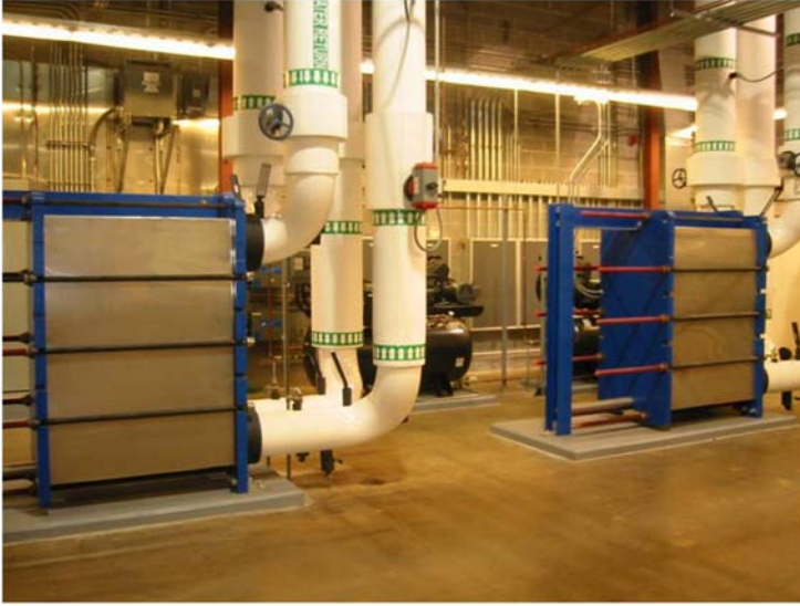
Figure 2.11 Insulated plate and frame heat exchangers.
