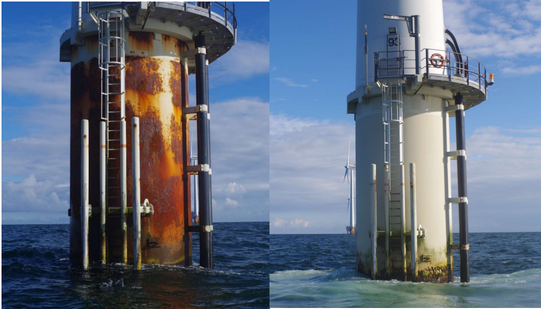
Figure 9. Horns Rev 14-year coating comparison, left: 350 \mu\text{m} ; right: 1000 \mu\text{m} (from Weinell 2017)
