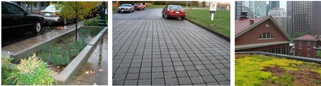
Figure 2a, b, and c: Examples of Green Infrastructure. From left to right: a planter box (bioretention), permeable pavers, and a green roof. (Source: US EPA, 2015b.)
