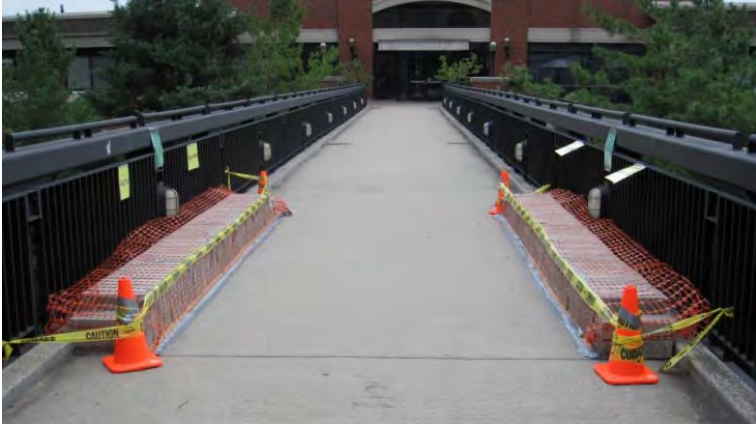
Figure 4. Concrete blocks loaded on footbridge's deck for three days.
