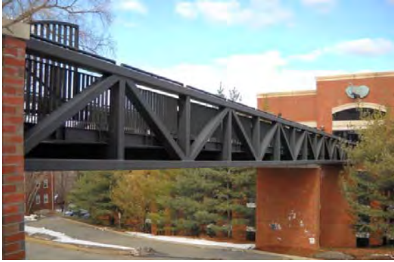
Figure 1. South view of the Dowling Hall Footbridge.
