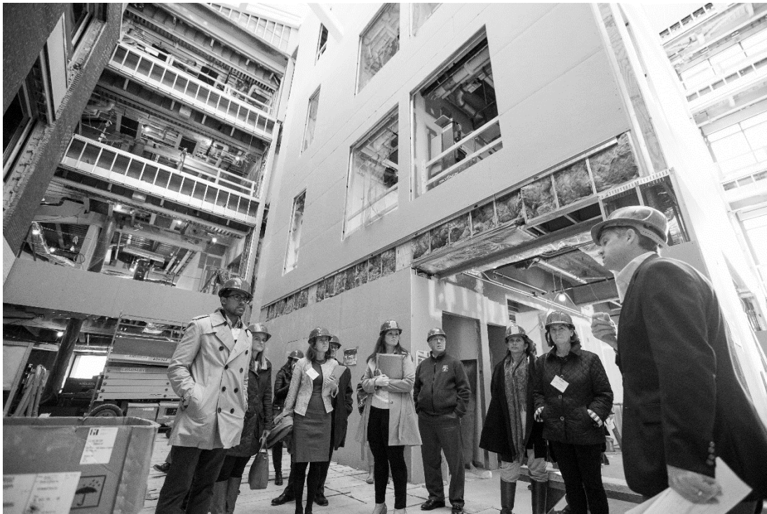
The new SEC building during a hardhat tour, November 12, 2016
