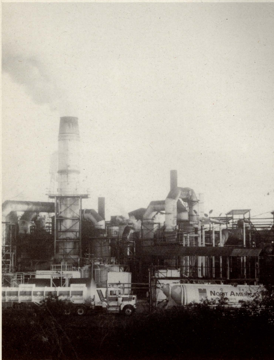
The Norit Americas activated carbon manufacturing plant in Marshall, Texas.
