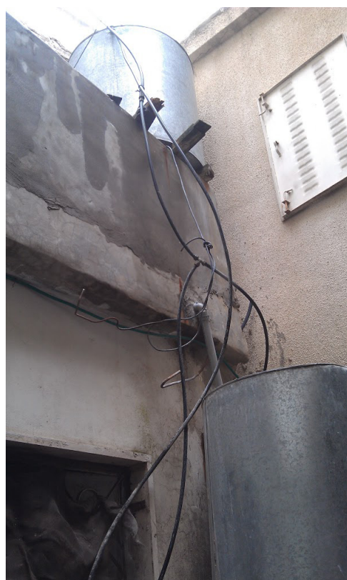
Figure 10 - Metal Rooftop Storage Tanks in Aida
