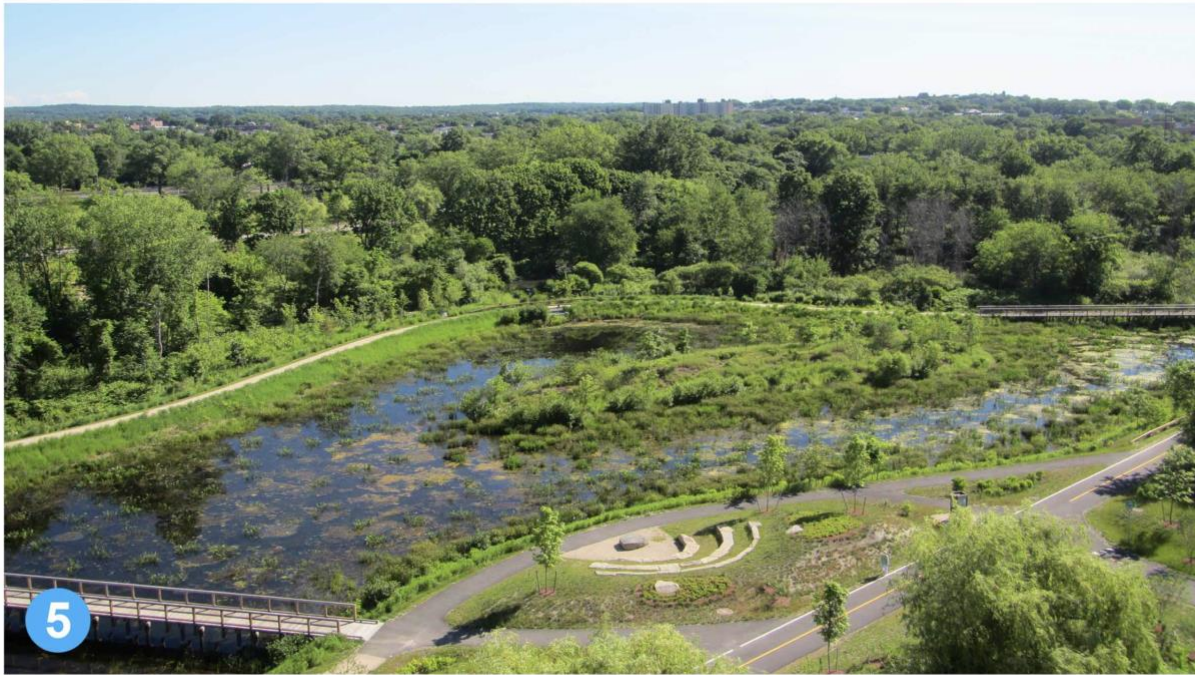
Upland peninsula at center of stormwater wetland basin (looking Northeast)
