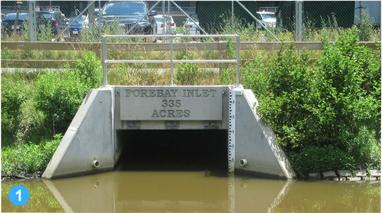
Inlet headwall from box culvert into wetland forebay
