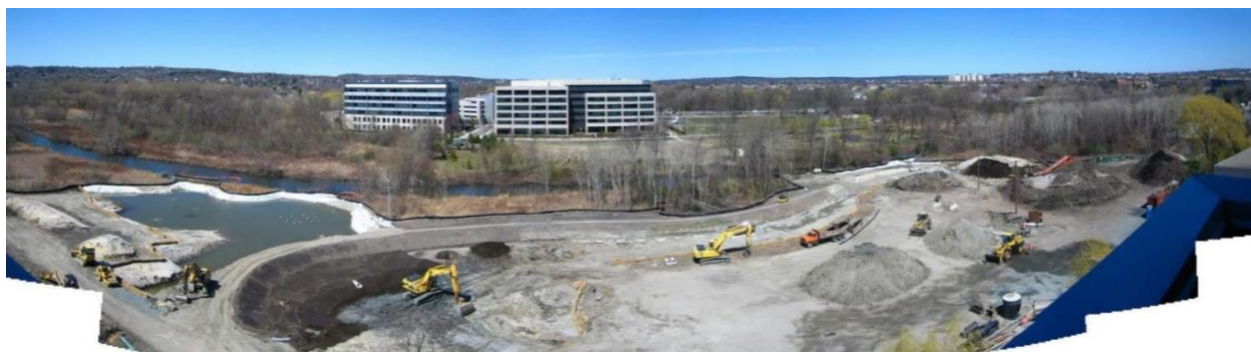
Figure 4.4 Initial Excavation of ASW. Source: Duke Bitsko
