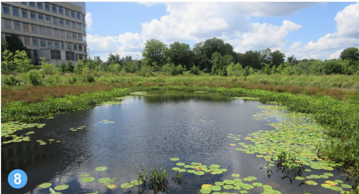
Permanent stormwater wetland pool (from timber overlook, looking West)
