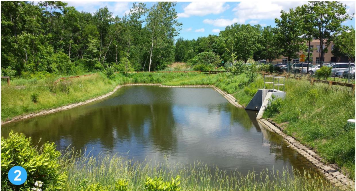
Wetland forebay (access ramp at rear, dewatering stand pipe on right)
