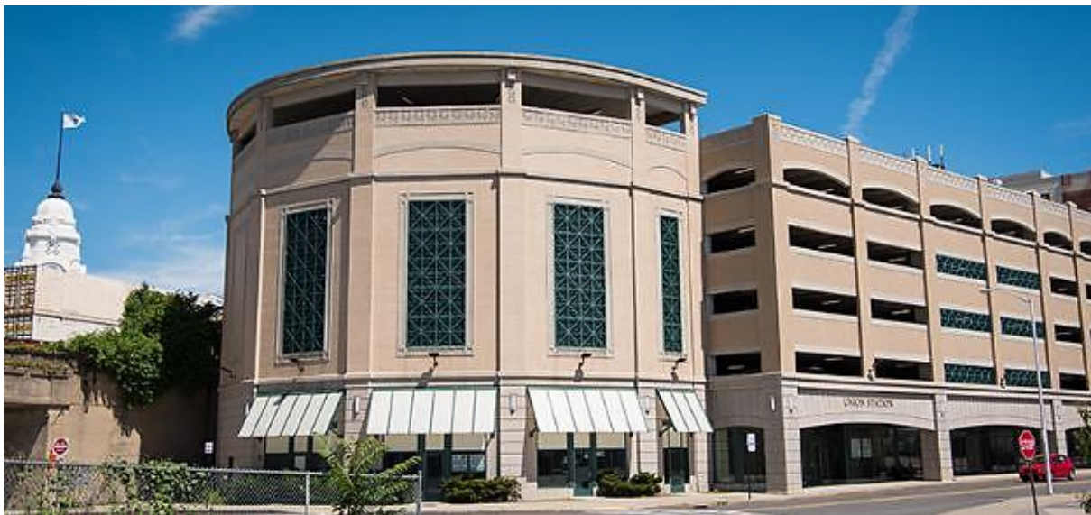
Figure 14. Worcester Union Station parking garage. Source: City of Worcester. https://www.worcesterma.gov/parking/municipal-garages
