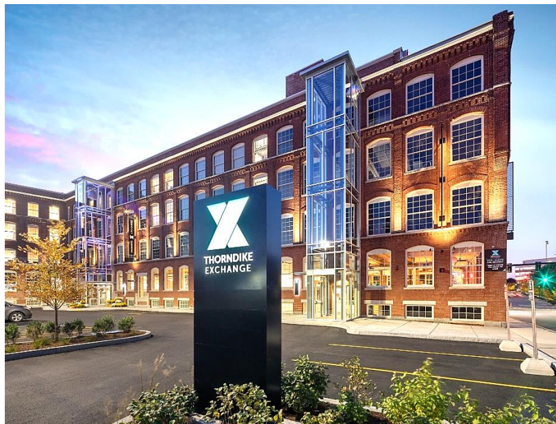
Figure 2. Thorndike Exchange, a mixed-use development next to Gallagher Terminal in Lowell. Source: BLDUP. https://www.bldup.com/posts/thorndike-exchange-sold-for-33-3-million-in-lowell .
