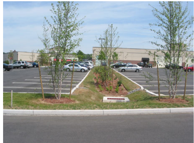
Figure 10. Bioretention System within Parking Lot Island
