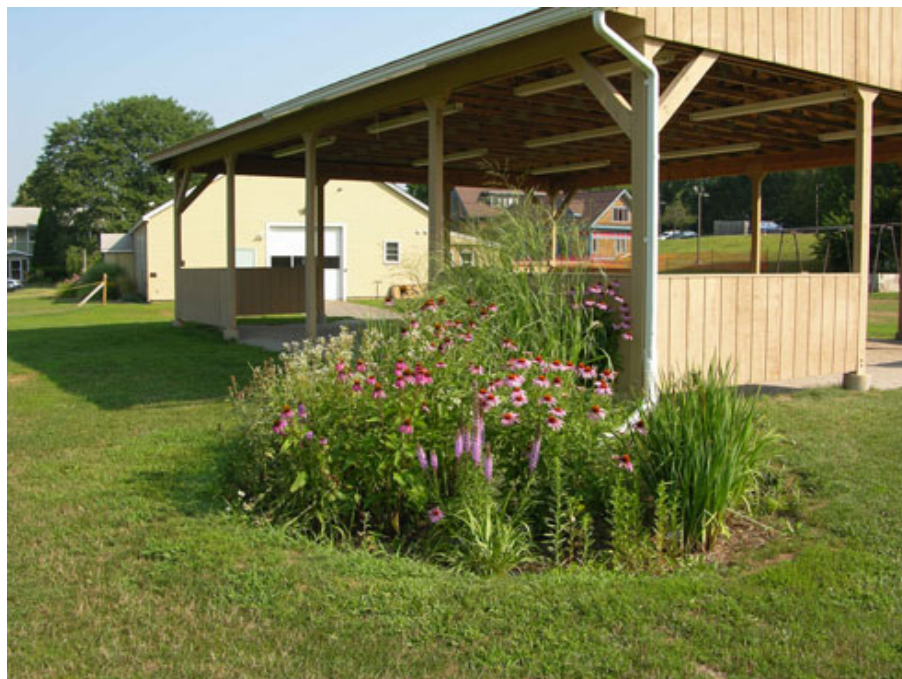
Figure 12. Rain Garden to Treat Rooftop Runoff
