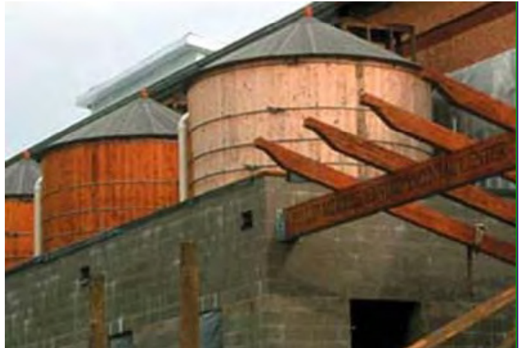
Figure 16. Example of Cisterns Used to Capture Commercial Rooftop Runoff
