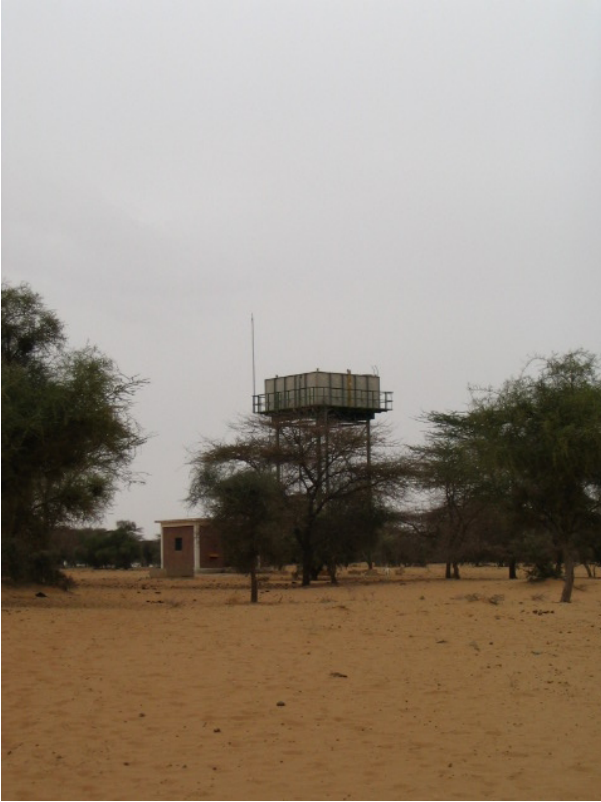
Figure 21: Storage Tank for Gravity Fed Reticulation System
