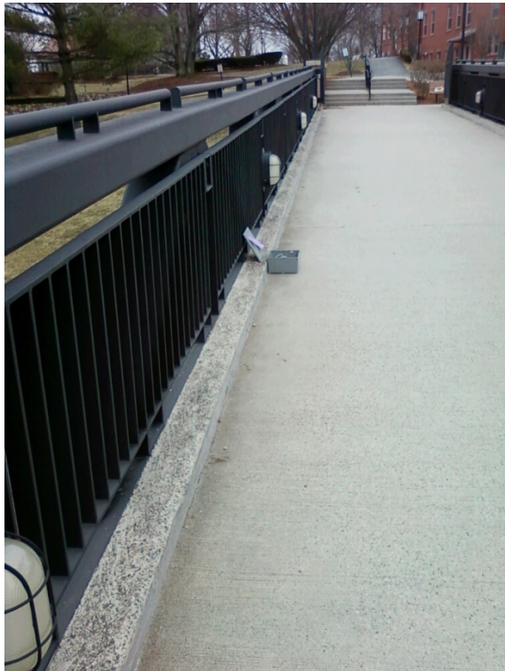
Figure 22: Setup on the Footbridge
