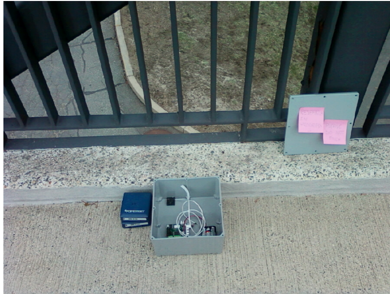
Figure 29: Narada Node in Test 2 (Left Side of the Bridge)
