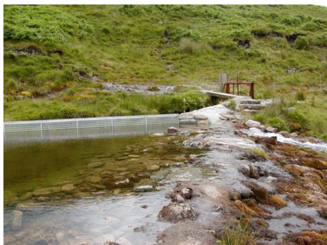
Figure 14: A passive mesh screen in Devon, UK. Source: United Kingdom Environment Agency.
