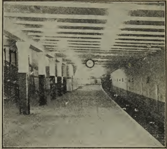
MILK STREET STATION, WASHINGTON STREET TUNNEL
