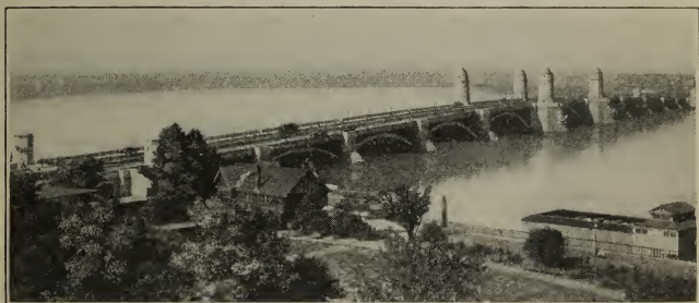
THE LONGFELLOW BRIDGE
