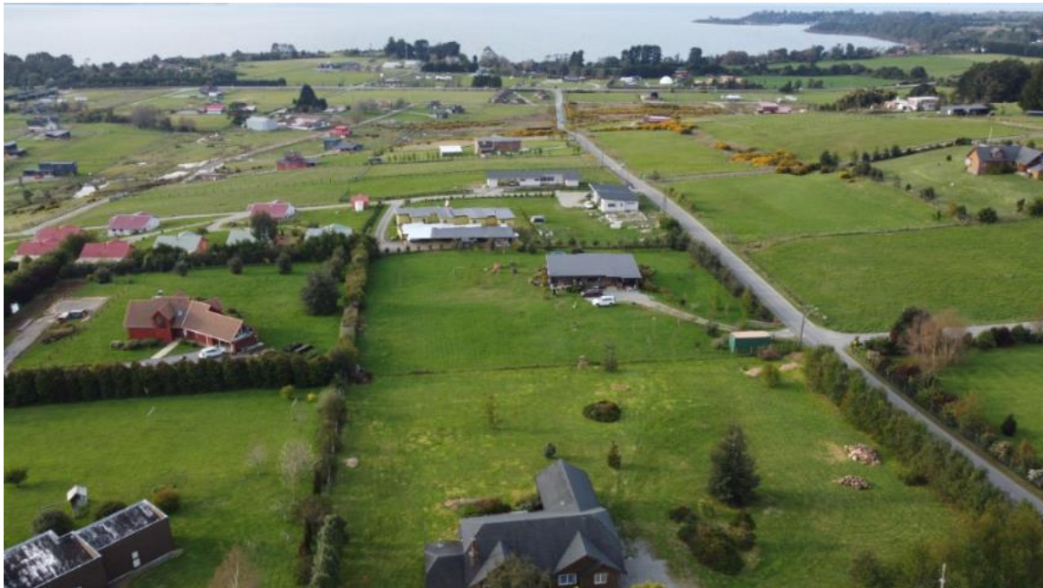
Figure 10: Example of a group of “parcelas de agrado” with built houses. Photo by El Mercurio Journal, 2023.
