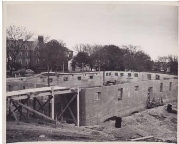
Image 3: Construction on New Henry Clay Jackson Gymnasium underway. 11
