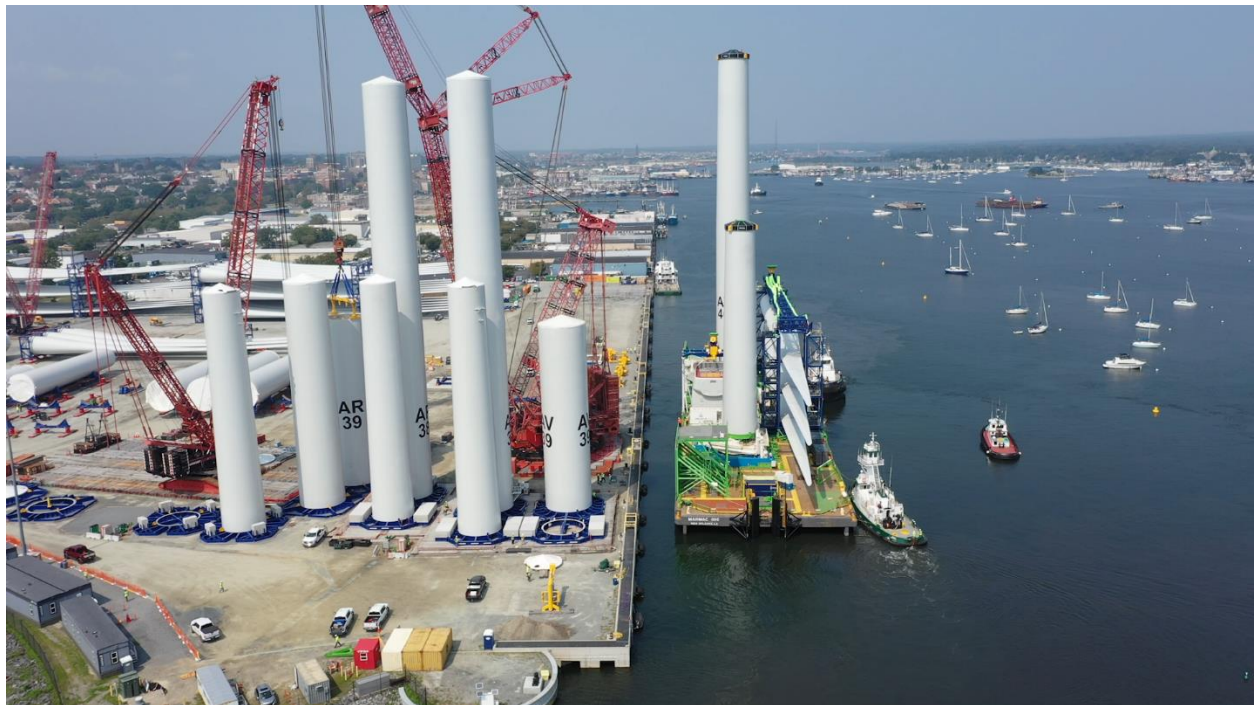
Figure 7. New Bedford Marine Commerce Terminal, used to stage Vineyard Wind 1. 152
