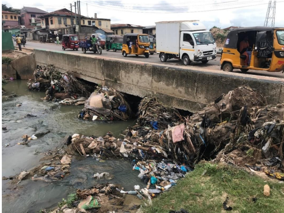
Figure 13. PW and MSW blocks storm drains leading to flooding during excessive rainfall, Kumasi, Ghana
