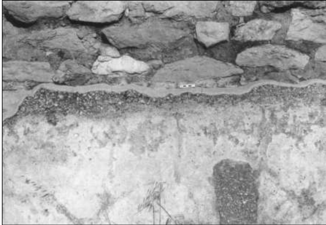
Figure 7: External face of the cisterns near the latrines at the Hadrianic baths. The crushed murex shells are evident in the mortar. 66
