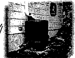
Runoff Retention Using Rainbarrel
