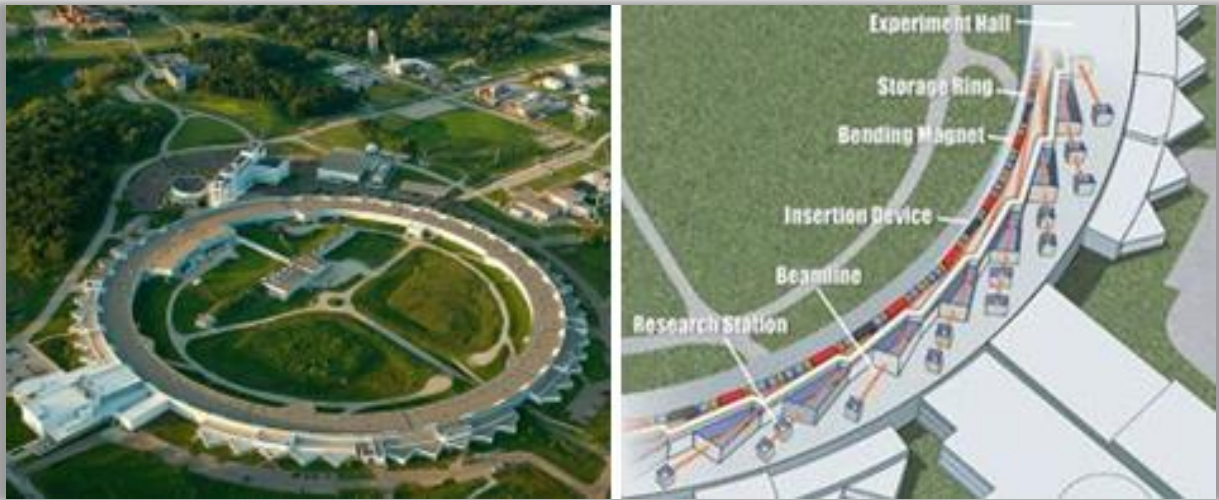
Figure 3-11: Synchrotron XRD located at the Argonne National Laboratory. Image reproduced from source: [46].
