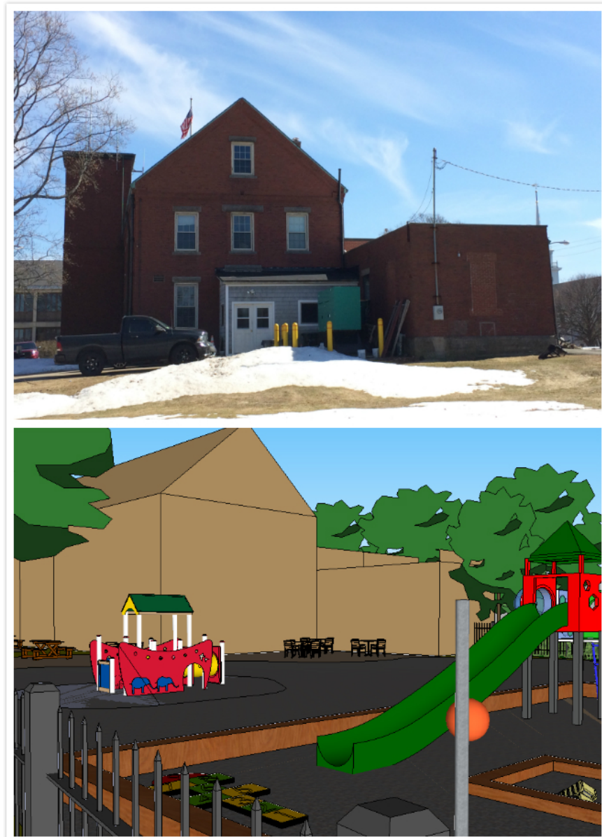
Figure 31: Before and after, playground behind renovated Fire Department building
