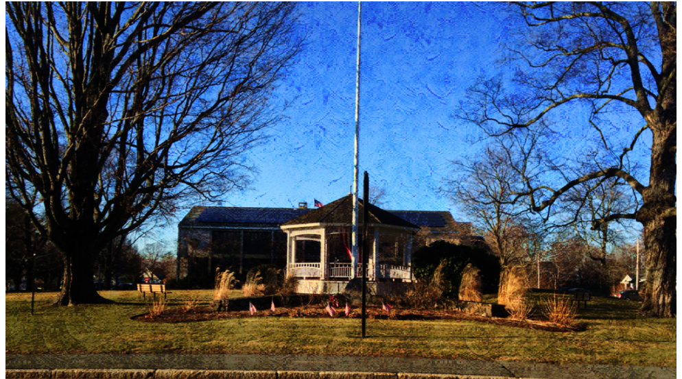
Looking across Canton Avenue, Gazebo in the foreground, Town Hall in the background
