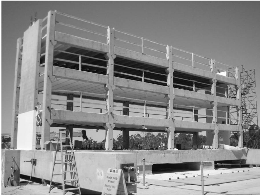
Figure 1 – South-East view of the tested structure.
