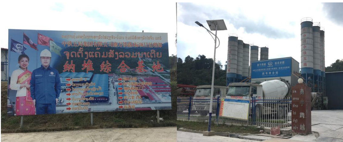
Photo6: CREC No5 Laos-China railways Boten-Vientiane company and material supply station
