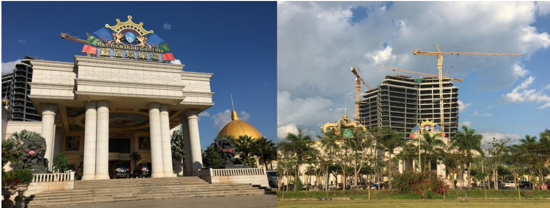
Photo9: The casino and the apartment house under construction behind (January 10, 2018)
