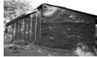
Mud-Adobe Dwelling with Iron Roof
