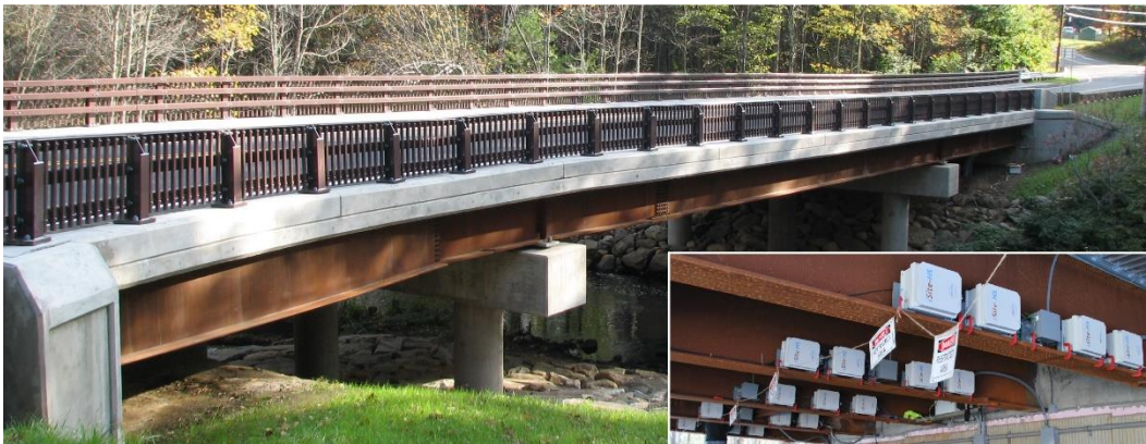
Fig. 1. Powder Mill Bridge and DAQ System
