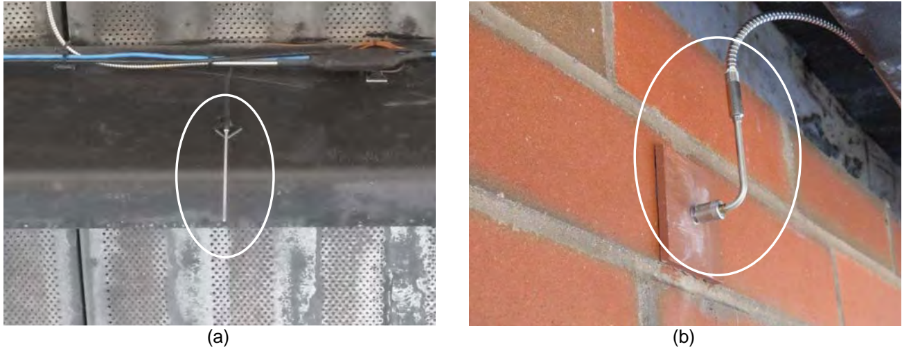
Figure 6. Installed Thermocouples: (a) air thermocouple A1, (b) concrete thermocouple C1
