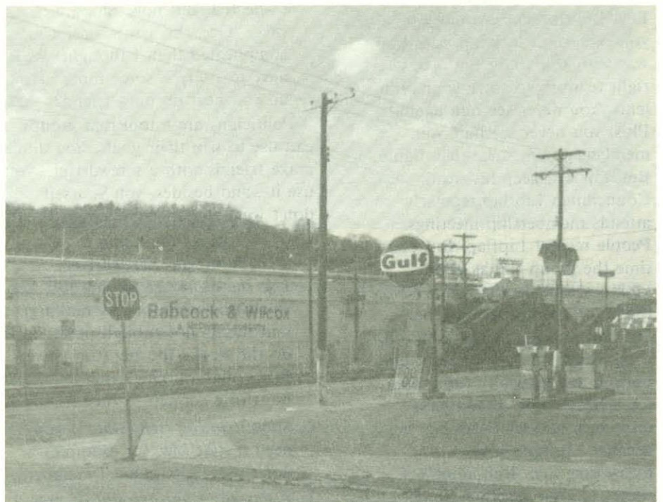
B&W's Apollo plant, taken from the corner of Cindee's street.
