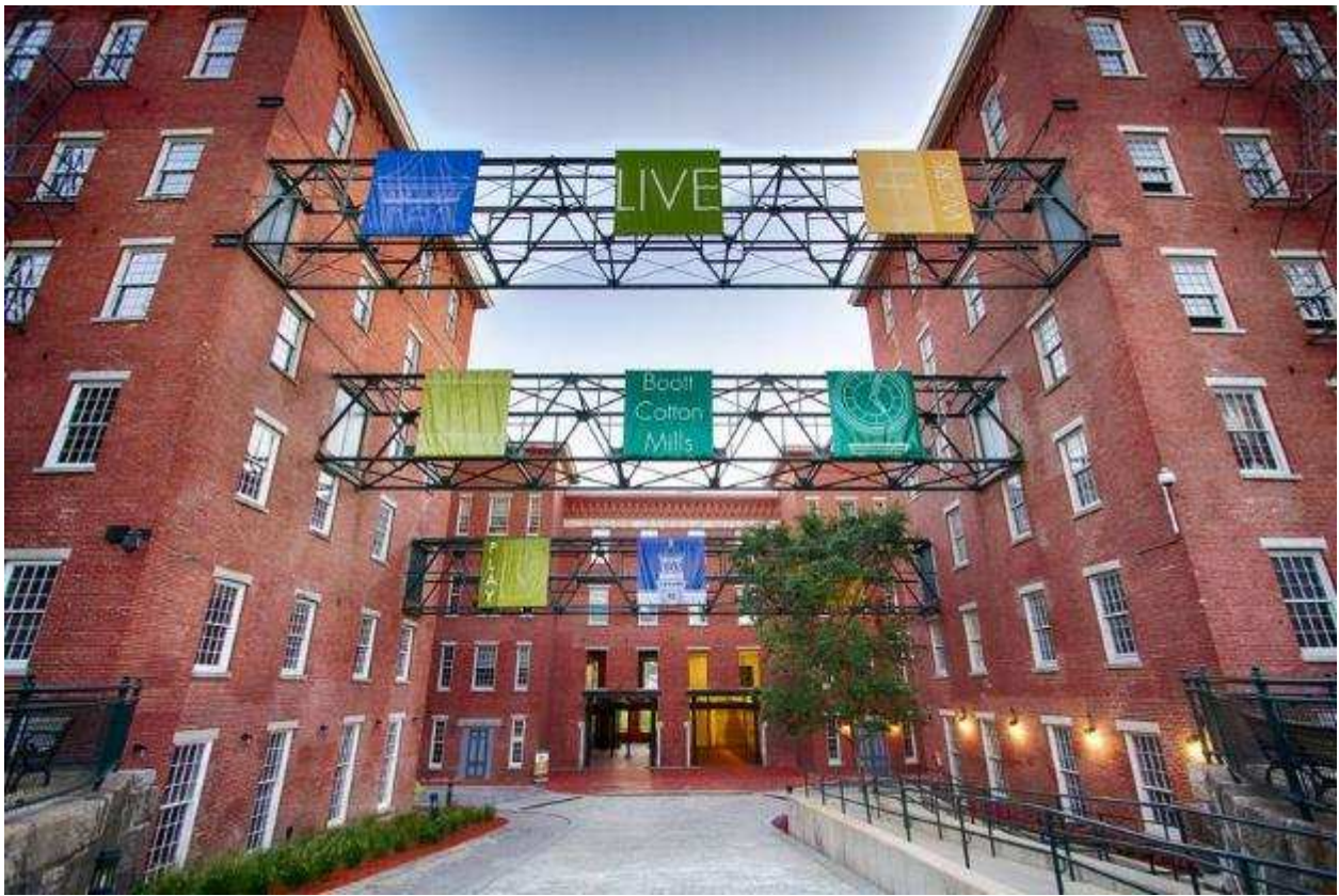
Figure 8: Entrance to Boott Mills Apartments Source: Winn Residential “Boott Mills,” Digital Image, Boott Mills, accessed March 10, 2019, https://www.boottmills.com/
