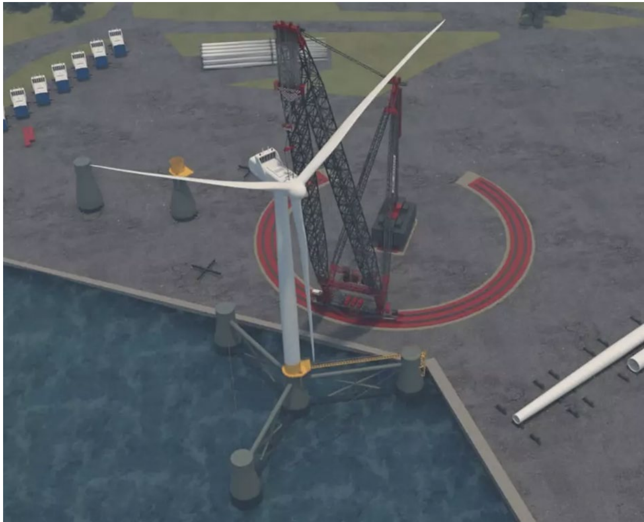
Figure 5: Mammoet SK6000 electric ring crane 19
