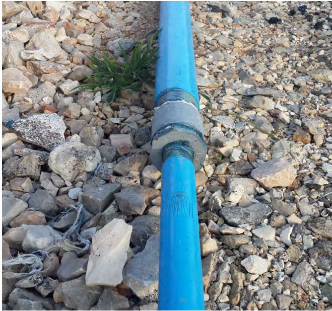
Figure 5. Variation in pipe size in Al-Walaja distribution system Source: Hiromi Hashimoto
