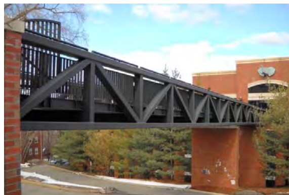
Figure 1. South view of Dowling Hall Footbridge
