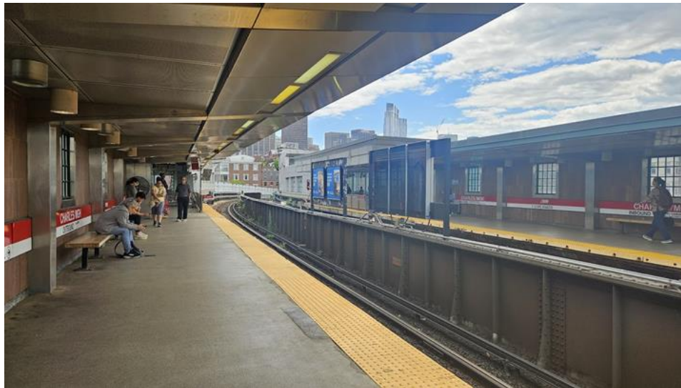
Figure 5.2: The Charles/MGH station
