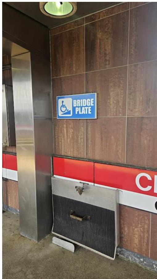
Figure 5.5: MBTA Bridge plate
