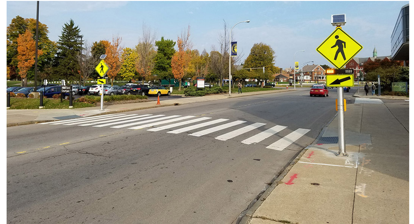
Figure 16: Rectangular Rapid Flashing Beacon at crosswalk (Carmanah)
