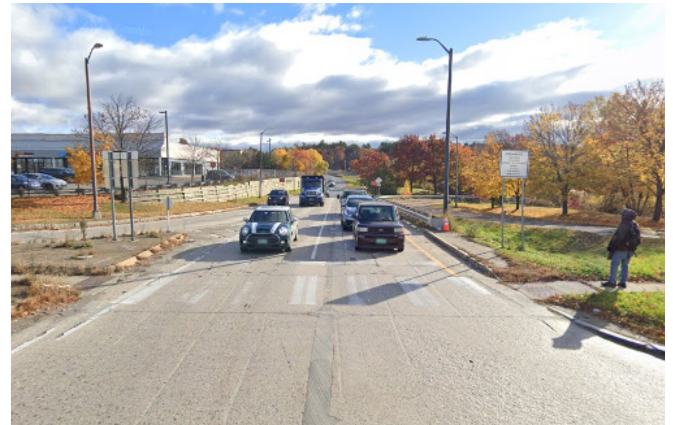
Figure 14: Uncontrolled pedestrian crossing across off ramp (Google Streetview)
