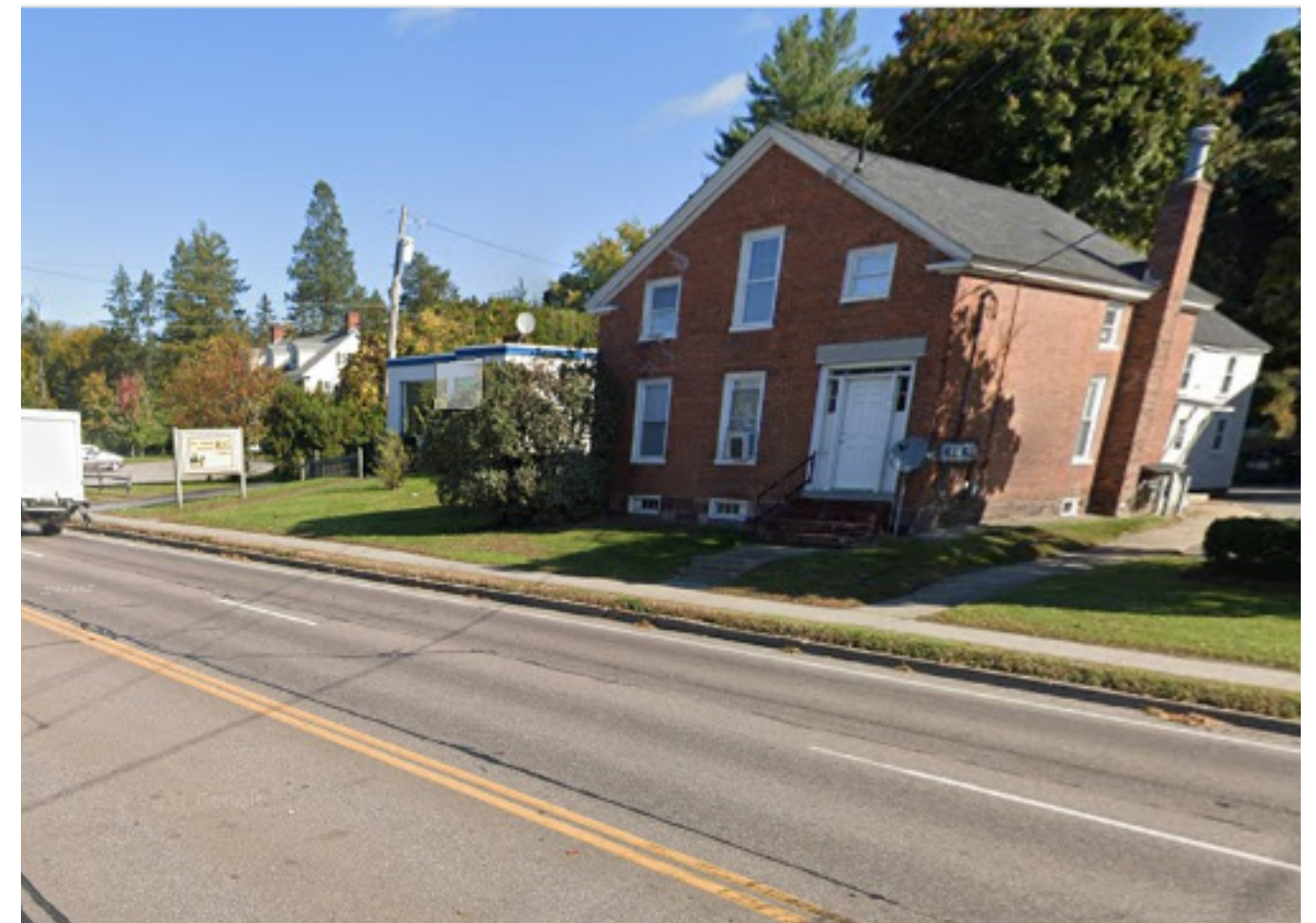
Figure 4: A historic street facing structure on Shelburne Road (Google Maps)
