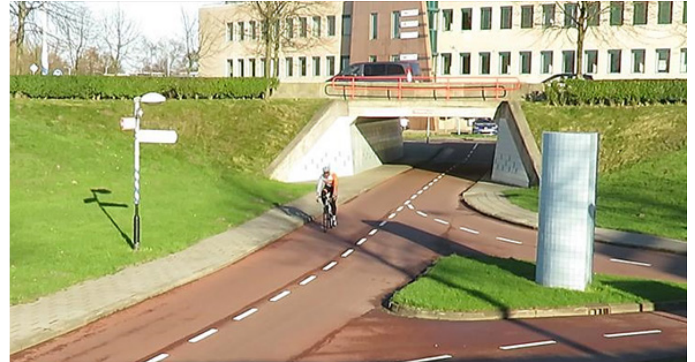
Figure 19: Bicycle Underpass - Netherlands.
