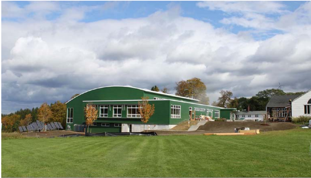
Putney School Field House, Putney, VT (MacLay Architects, 2010, "The Putney School Field House")
